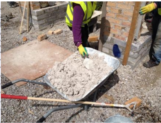
One of the hot lime mortar mixes ready for use.
