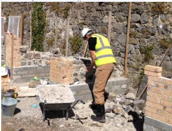
One of the hot lime mortar mixes ready for use.
