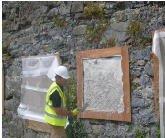
Preparing the harling test panels
