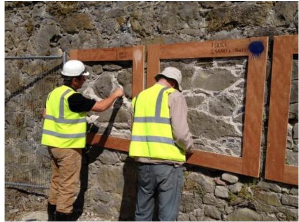
Pointing of the rubble wall panels.
