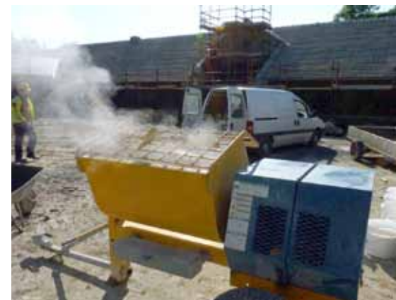
Larger quantities of mortar require the use of a machine.
