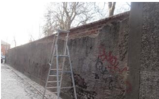
Boundary wall to St. Catherine's graveyard prior to re-harling.
