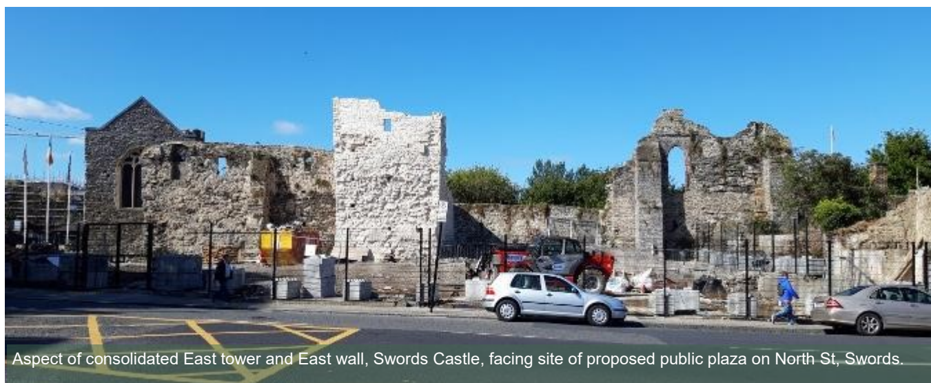
North/East elevation of tower after shelter coat.
