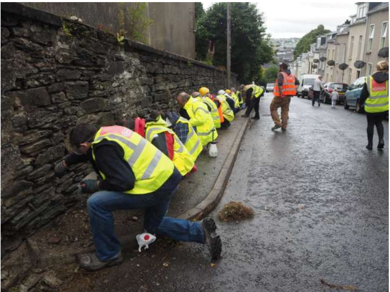
Volunteers re-pointing a garden wall during the 2018 Working Party in Derry
