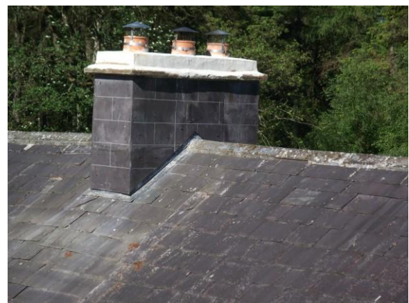
Restoration of chimney at Augnagaddy House Ramelton, using reclaimed Bangor Blue Slates to match existing – Tir Conall Restoration/ Sean Brogan.
