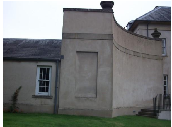
New Lime render comprising of carefully selected lime, aggregates and oxide pigments to match existing render – Oakfield, Raphoe, Co. Donegal. By Sean Brogan.
