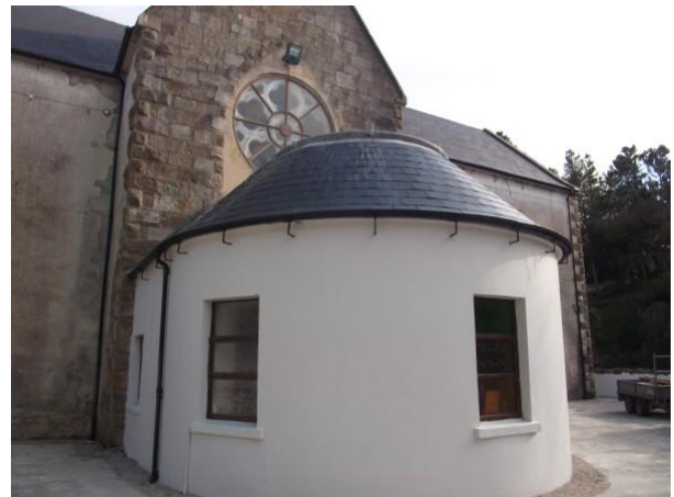
Radius cast iron guttering and lime render to Old Church at Derrybeg Co. Donegal – Sean Brogan
