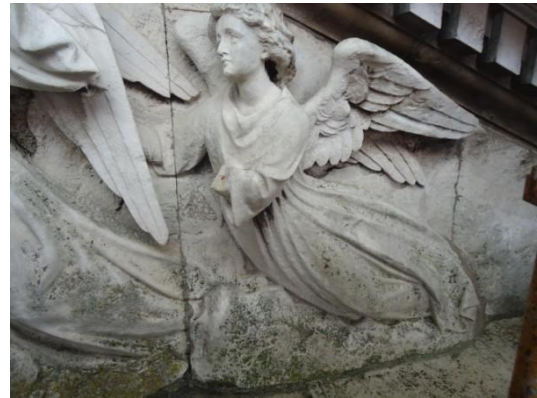
Above – Before work commenced with Angels hand missing, facial features eroded, inappropriate cement re-pairs, ponding of water in bas-relief, erosion and decay widespread.
