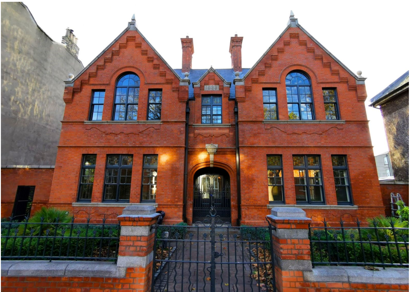
No.5 Northumberland Road on completion of works.
