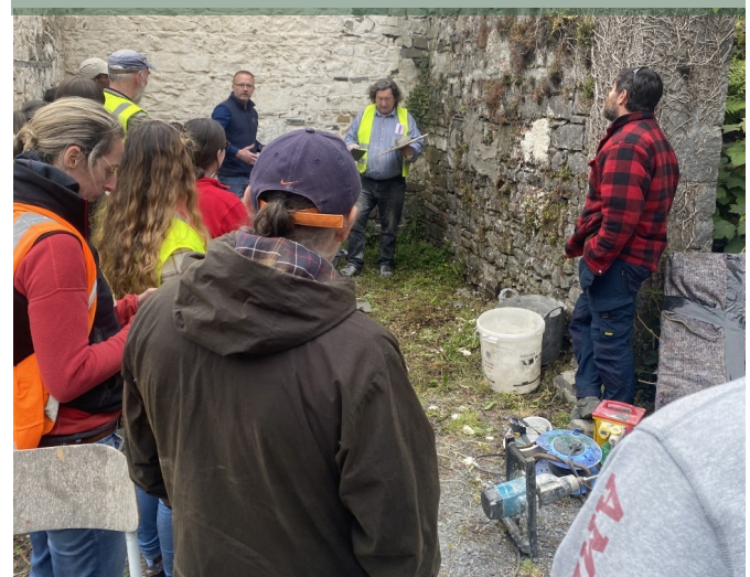
Henry Thompson (BLFI Board Member) demonstrating the application of insulating lime renders.
