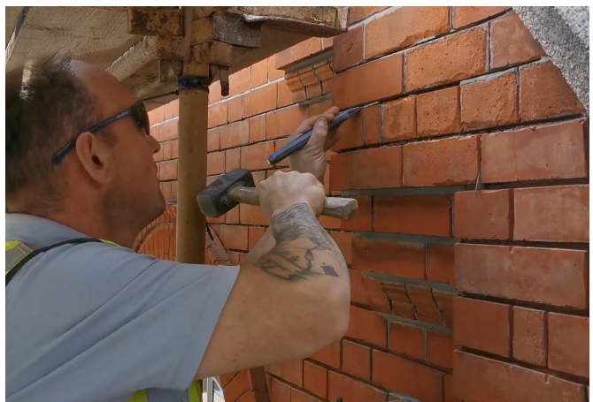
Raking out of inappropriate cement-based mortars.
