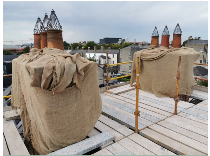
Protection of lime works to chimney stacks.
