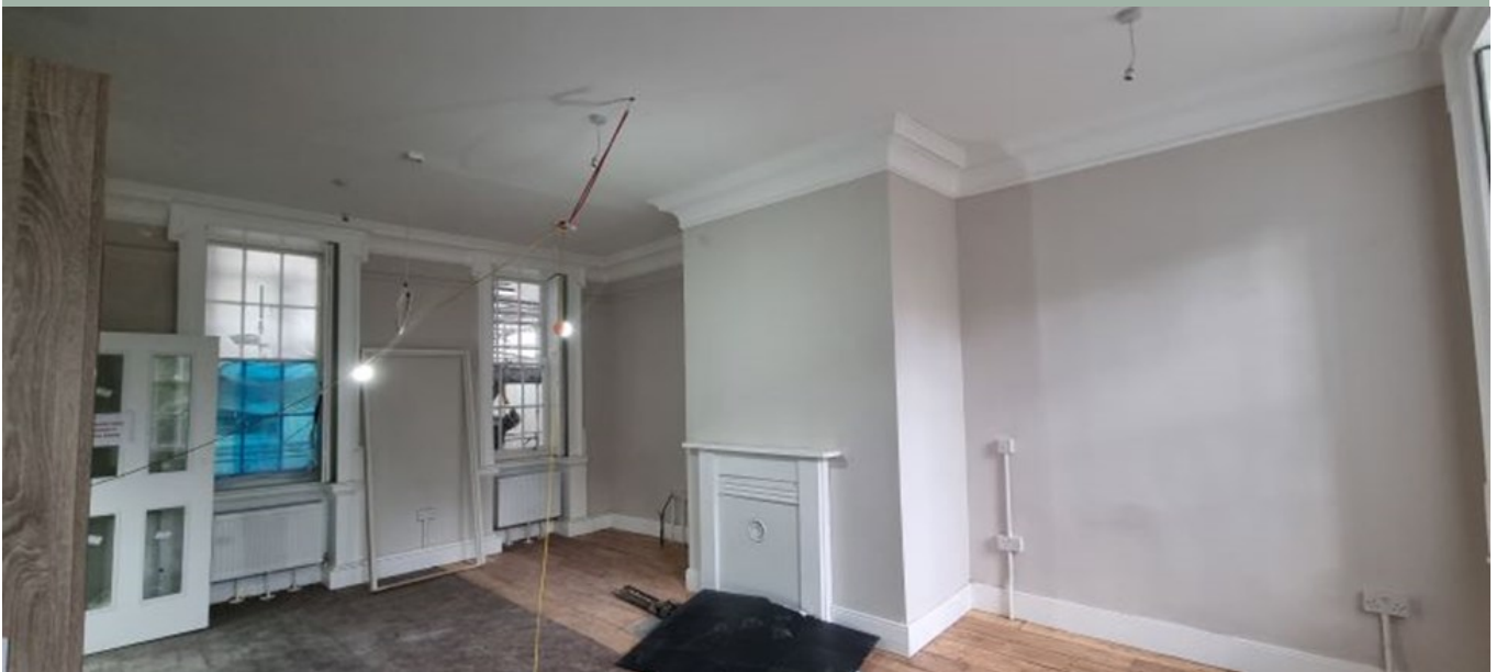
Completion of plaster conservation works to the Rubrics, Trinity College.
