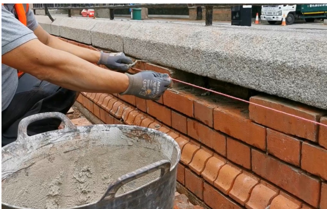
Replacement of irreparably damaged brick.
