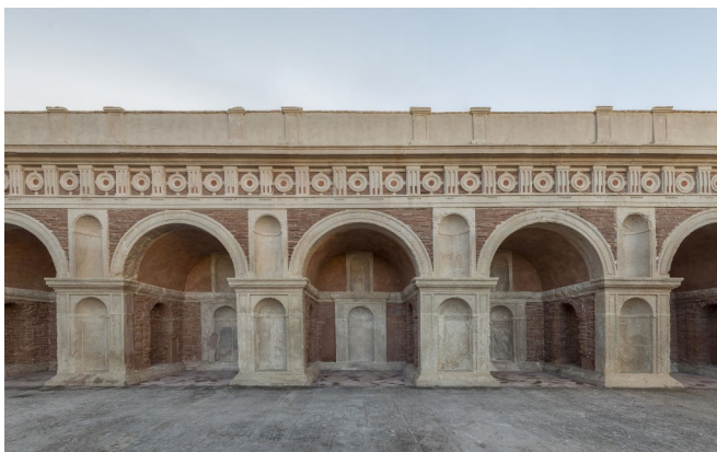
Renaissance "loggia" on completion of works.
