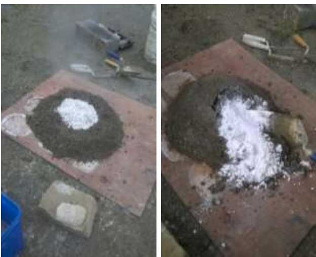
Mixing mortar on boards
