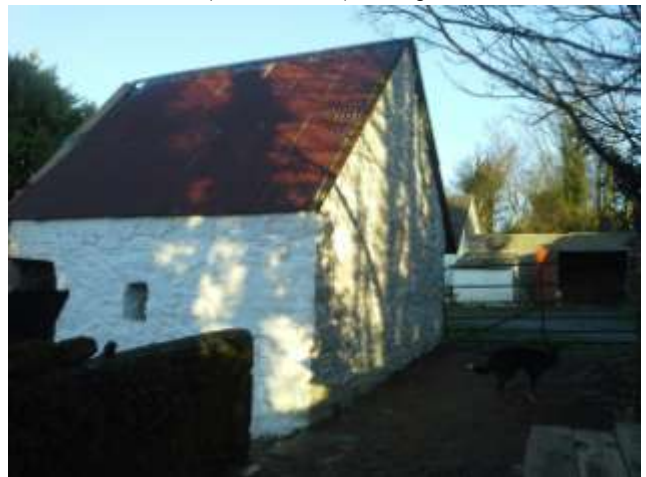
Lime wash on completion, 6:1 water to lime putty
