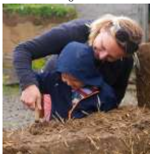
Cob repair, Laois
