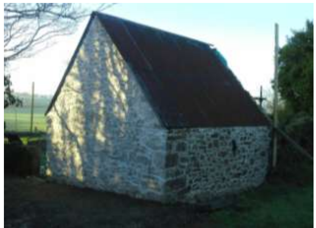
Rear view on completion of re-pointing
