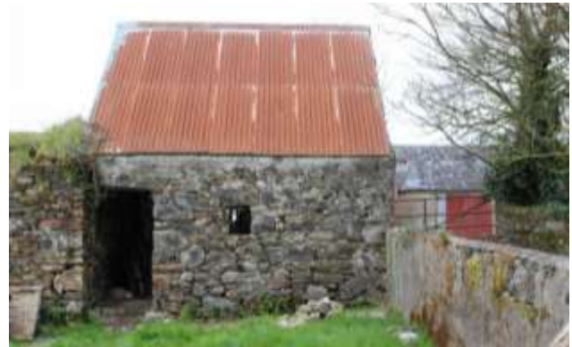
The 'Sheep Shed 'before the works commenced
