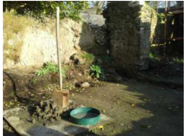
Hand-crushing and sieving earth to powdery clay
