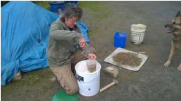
Preparing dry-mix on boards
