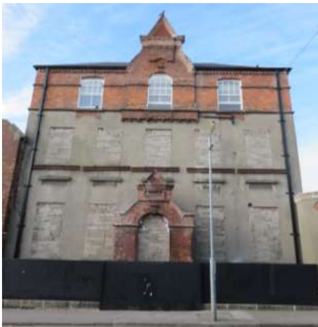
Principal (North) elevation prior to façade restoration.
