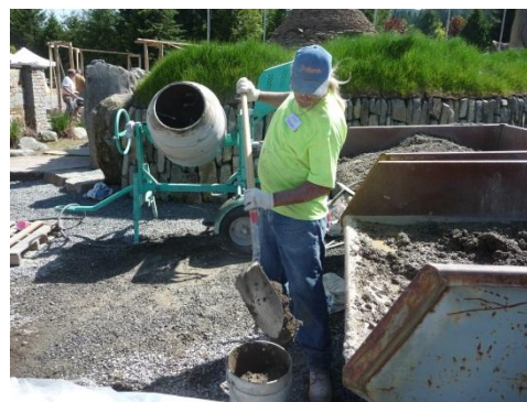
Batching wet clay from a skip in to a bucket
