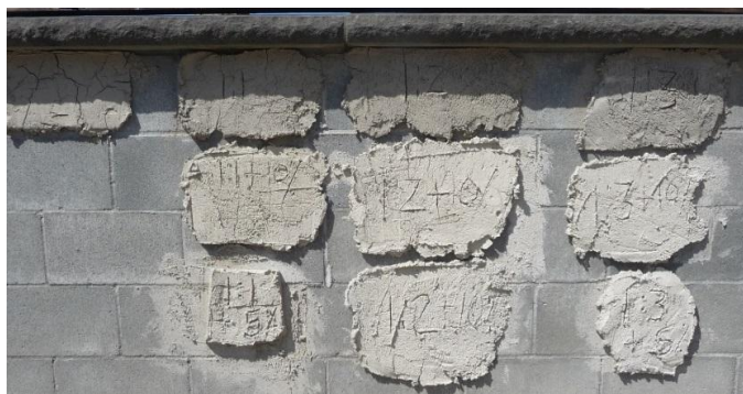
Test panels showing various samples of clay, clay and sand and clay, sand and quicklime mixes
