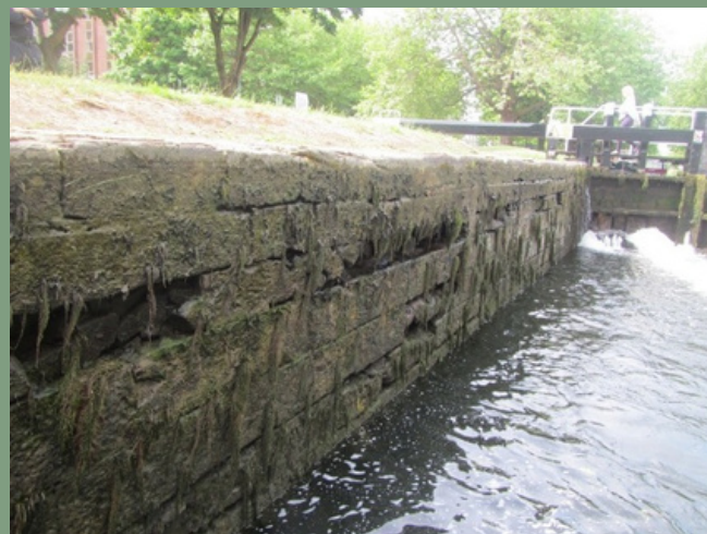
Rows 3 and 6 in particular had significant damage to the Calp Masonry
