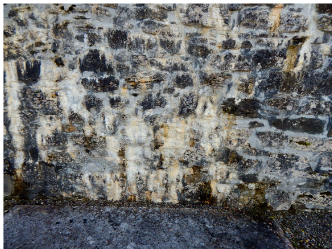
Cong Abbey, Co. Galway. Formerly collapsed wall rebuilt and pointed with NHL 3.5-bound mortar and block-laying sand 2014. The wallhead was well protected, but water is suspected of building up from ground level upwards. Image: Author
