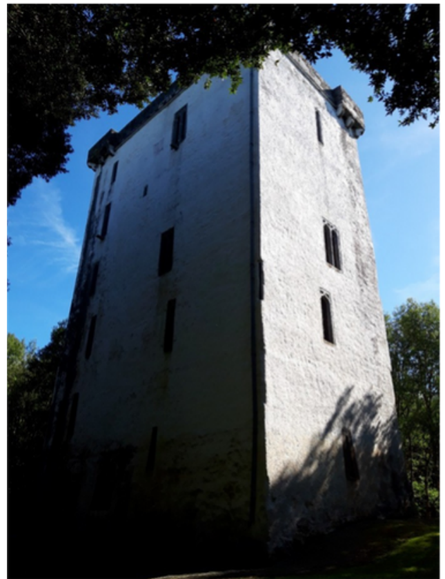
Ardamlivian castle, Co. Galway. Coated with lime harl and limewash in 2006 by the OPW. Image: Author
