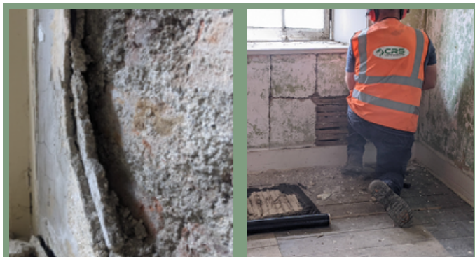
Fig 2. Plaster on a rubble stone wall during removal (a) removal of sections of lath-and-plaster (b)
