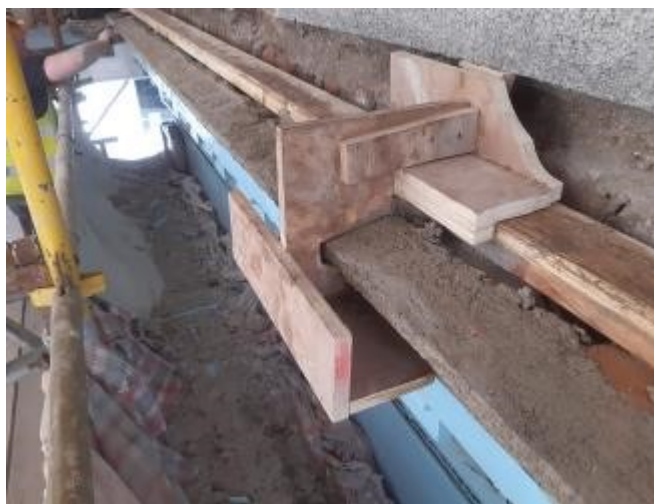
Horse for running cornice repairs.
