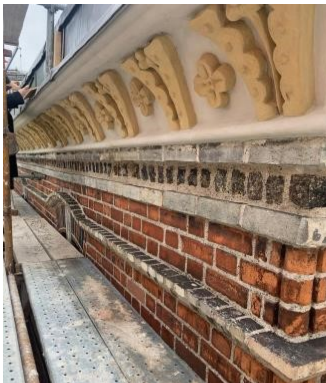
Repair works to cornice at Trinity Street and St. Andrew's Street, Dublin.
