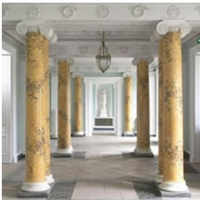
Exquisite scagliola columns flanking the entrance hall at Fota House, Cork.
