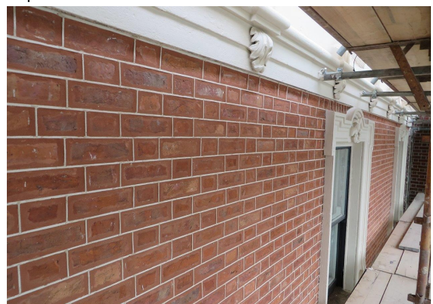
Wigged re-point above. Technique diagram below.
