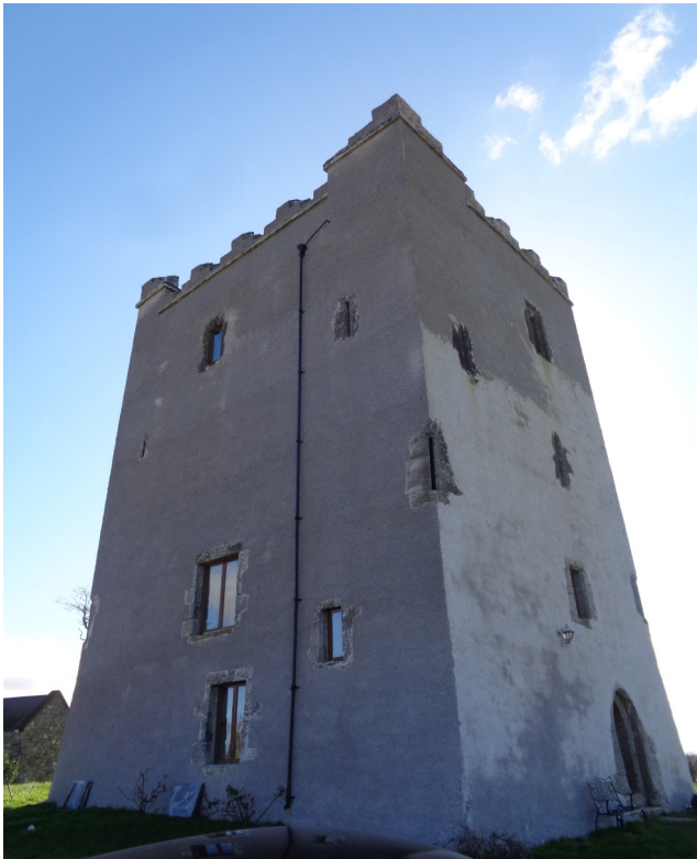
Photographs of the completed external render above & below the improved internal walls and main door surround detail
