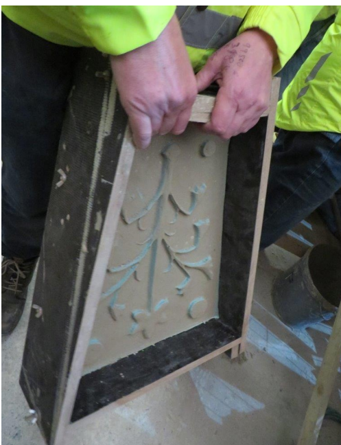
Left: Moulds for Roman cement casts. Above: Turned out Roman cement casts, drying before being prepared for fixing
