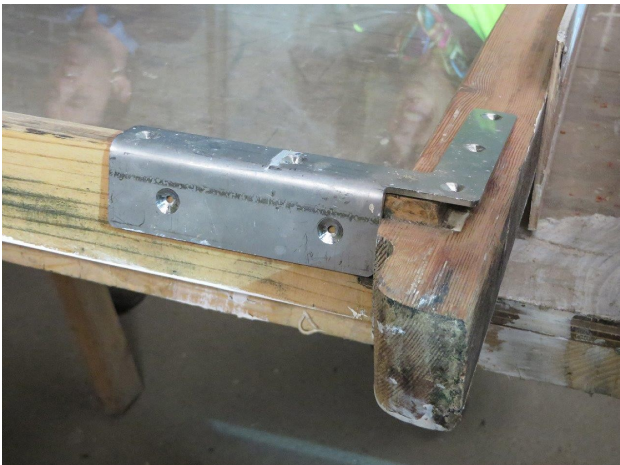
Sash repair bracket for timber joints
