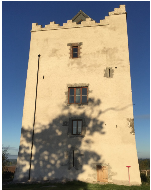
Photographs of the completed external render above & below the improved internal walls and main door surround detail
