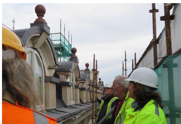
Repaired structure and lead work of the dormer windows
