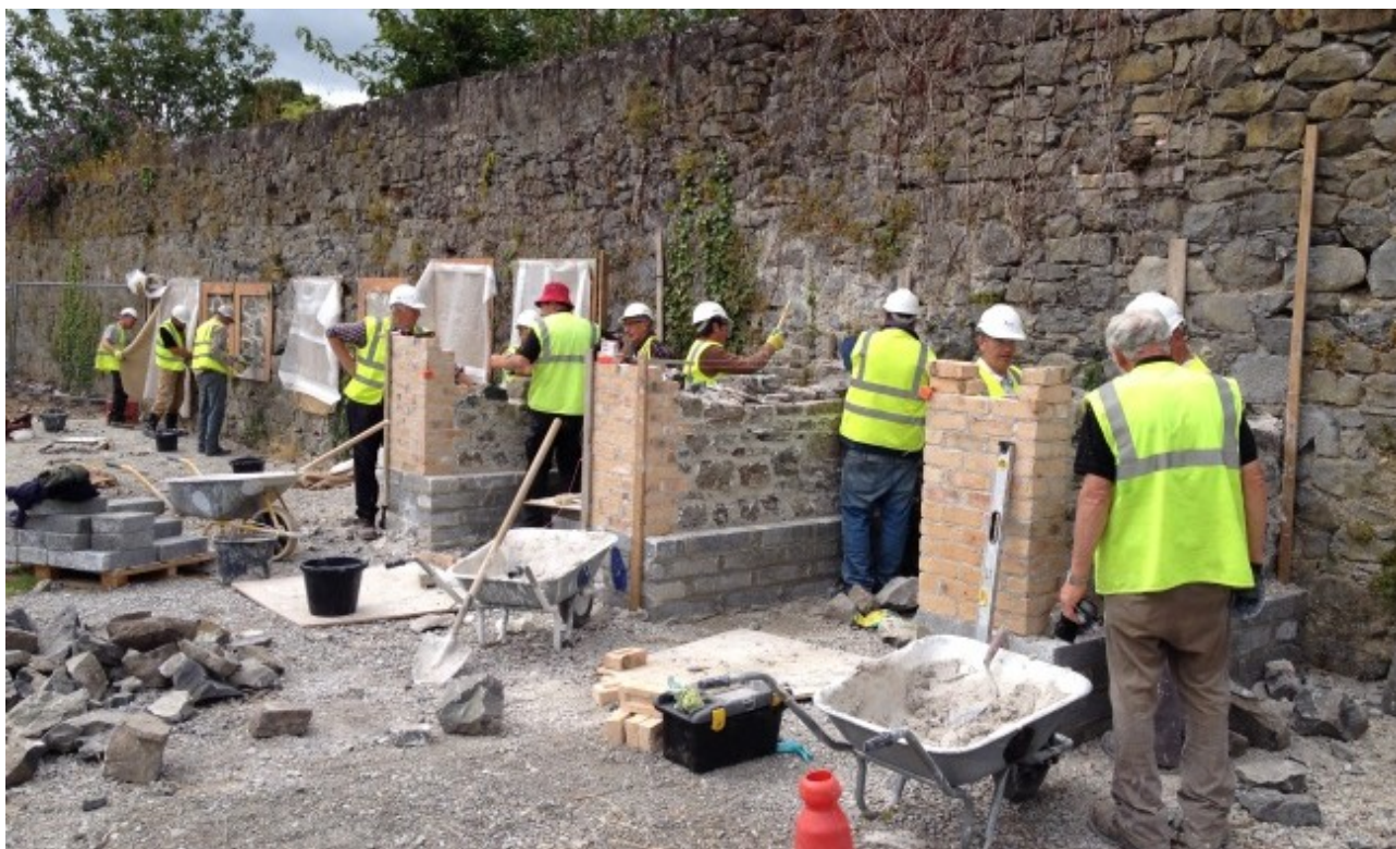
Construction of test walls
