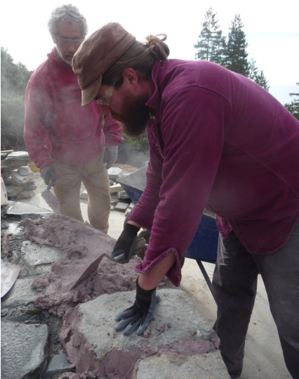
Steam rising from hot-lime mortar
