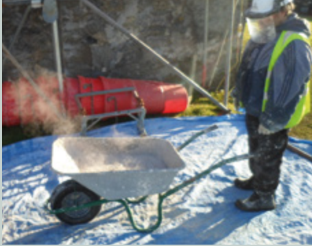
Fig. 8 Hot-mixed lime mortar ready for use on site. © Shetland Amenity Trust
