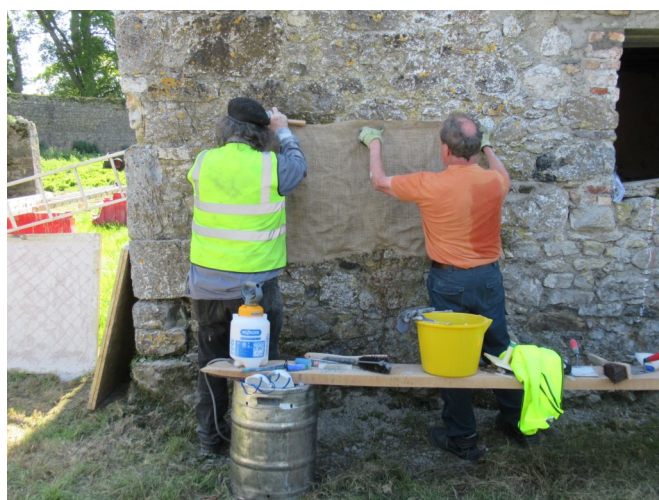
Henry Thompson demonstrating the protection of lime mortar.
