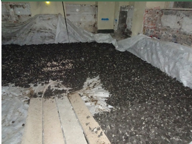
FGA being installed over a geotextile membrane.
